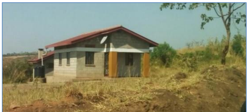
Photograph 7-6: Typical replacement house that will be built for resettled families on the Buhuka Flats
