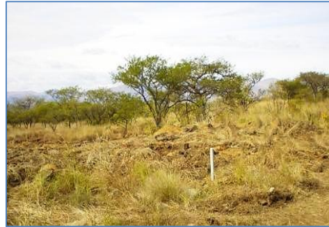
Reinstated surface with pipeline centreline marker
