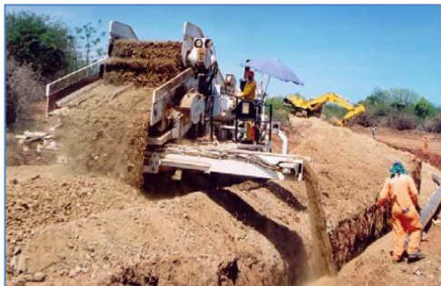
Screening plant backfilling the trench
