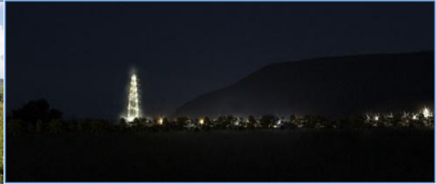
Figure 7-8: Night time view of Drilling Rig 1, the permanent camp and the production facility after tree screening
