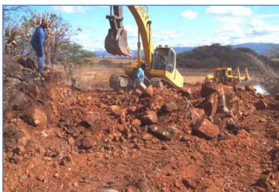
Clearing and grubbing
