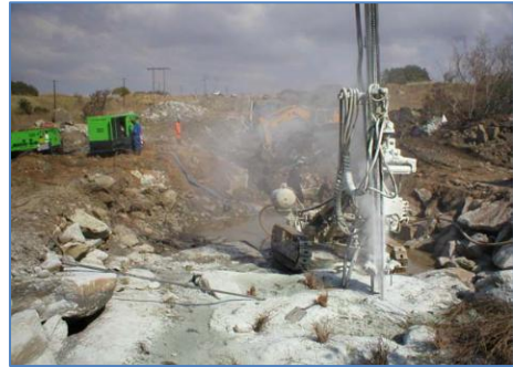
Blasting in rocky areas
