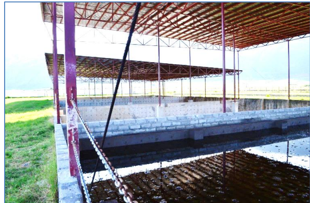
Photograph 7-2: Current arrangements for the temporary storage of drilling waste on the well pads. This design may be modified for the production wells to improve dewatering and re-use of drilling fluids.
