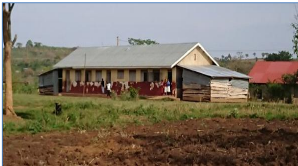
Photograph 6-29: A school along the pipeline route
