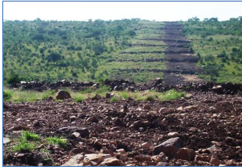
Reinstated surface with drainage berms
