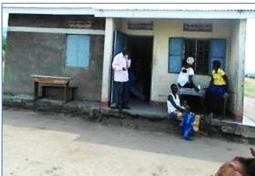
Photograph 6-20: Buhuka Health Centre III
