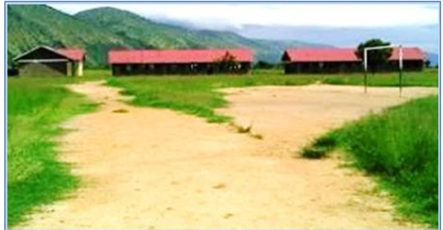
Photograph 6-22: Buhuka Primary School
