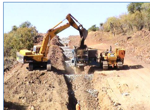
Trench breakers on steep slopes
