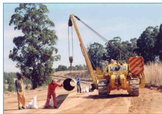
Pipe string along the construction right of way
