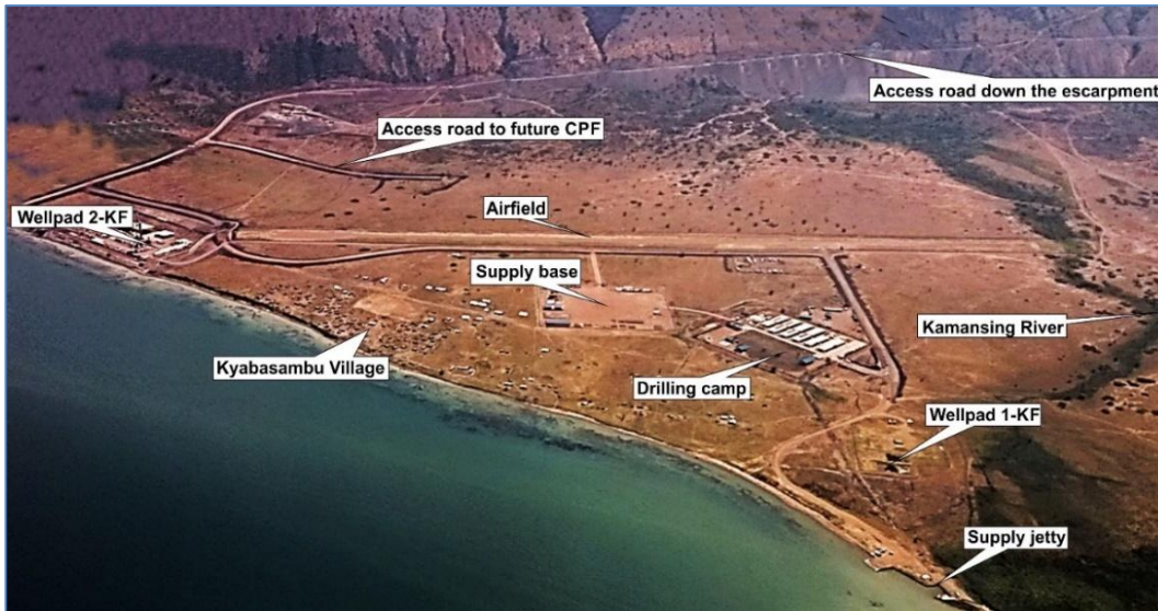
Figure 2-1: Overview of the existing main project infrastructure
