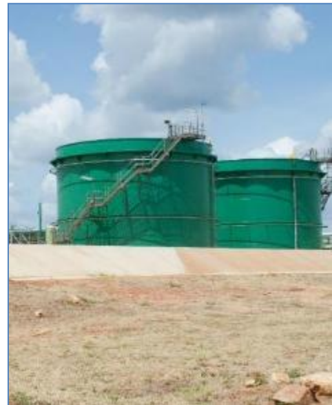
Photograph 2-4: Typical stabilised oil floating roof storage tanks
