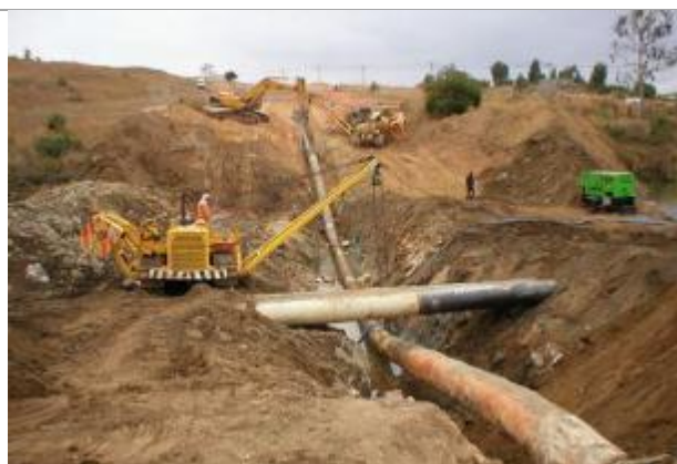
River crossing (note flume pipes)
