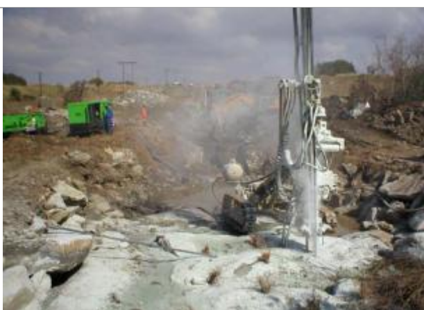
Blasting in rocky areas
