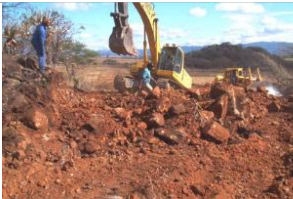
Clearing and grubbing
