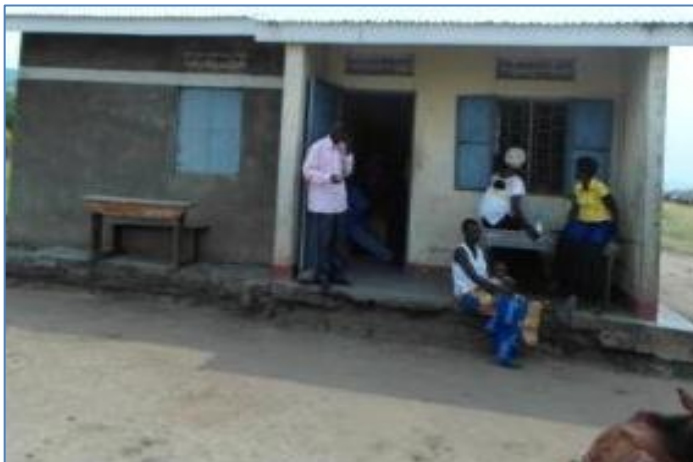
Photograph 6-27: Buhuka Health Centre III
