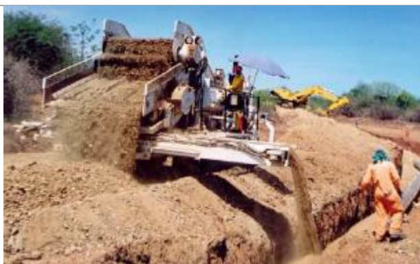
Screening plant backfilling the trench
