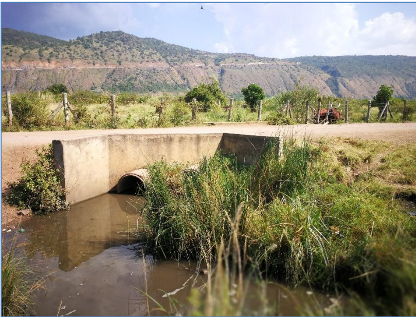
Photograph 8-3: Road culvert across the main channel of the Kamansiniga River
