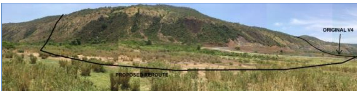
Figure 16-2: Kingfisher feeder pipeline re-route near the CPF
