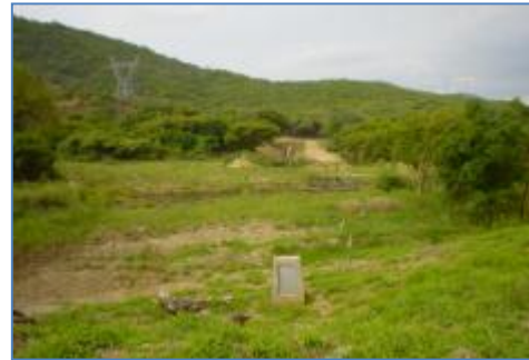
Photograph 2-3: CP Post along a pipeline route
