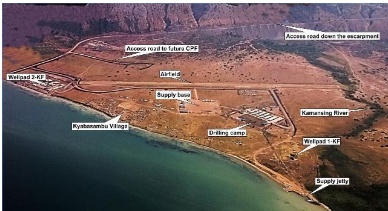
Figure 2-2: Overview of the existing main project infrastructure
