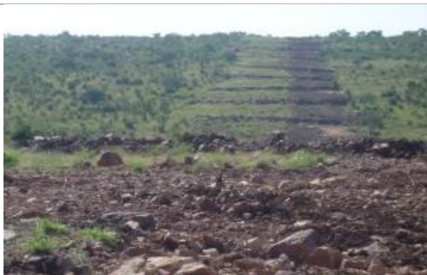
Reinstated surface with drainage berms
