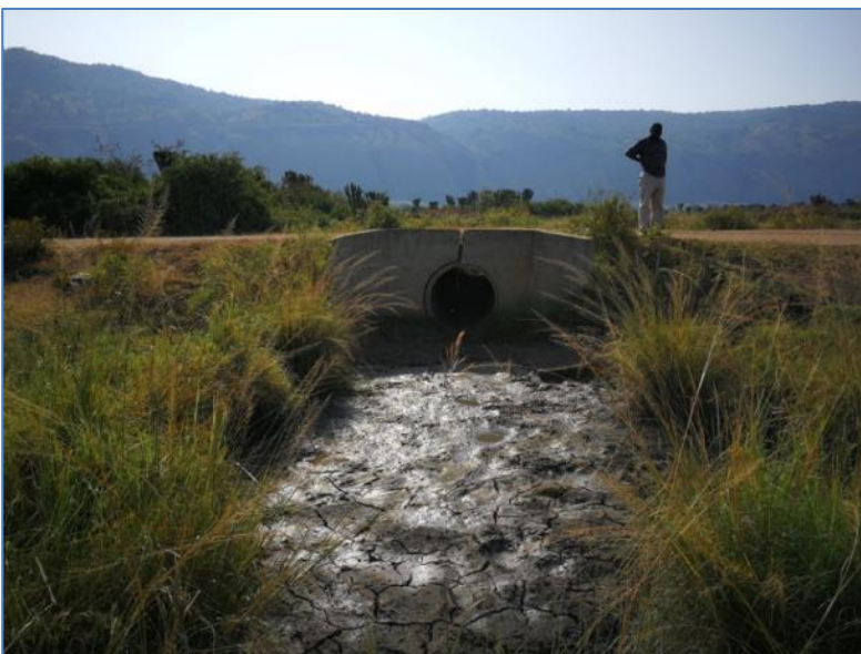
Photograph 8-4: Road culvert across the subsidiary channel of the Kamansiniga River
