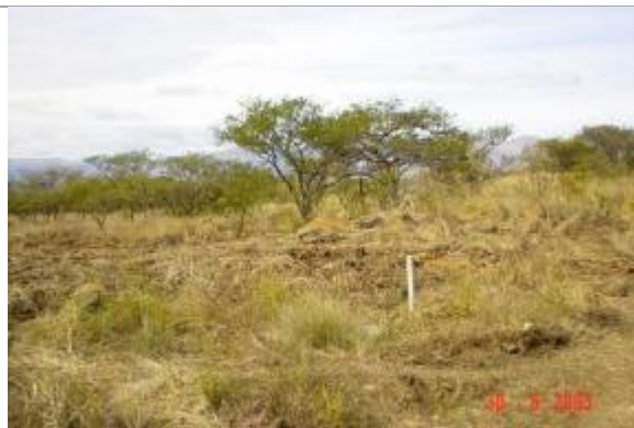
Reinstated surface with pipeline centreline marker
