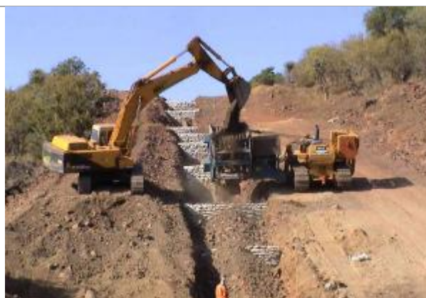
Trench breakers on steep slopes
