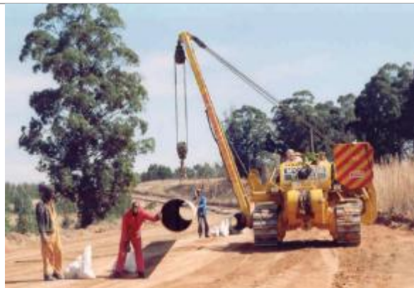
Pipe string along the RoW
