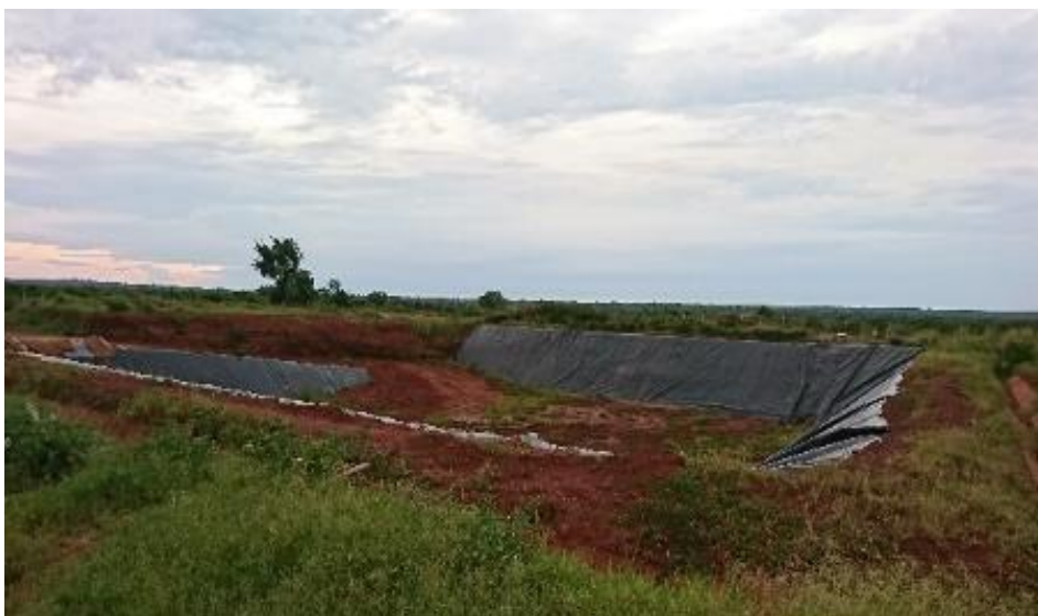
Figure 8: One of the Open Cells at the Luwero Landfill Site
