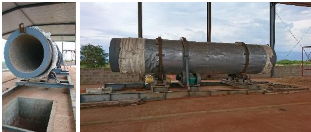
Figure 13: Dual-chamber Rotary Kiln under Construction at Luwero's Facility
