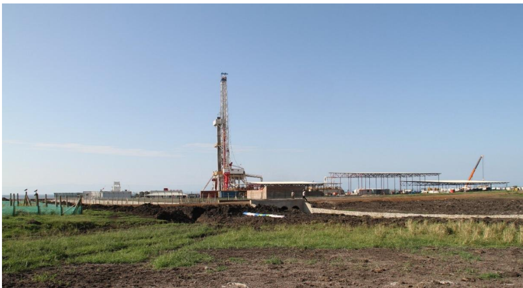
Figure 19: The well pad drill rig is the most visually intrusive element of the project
