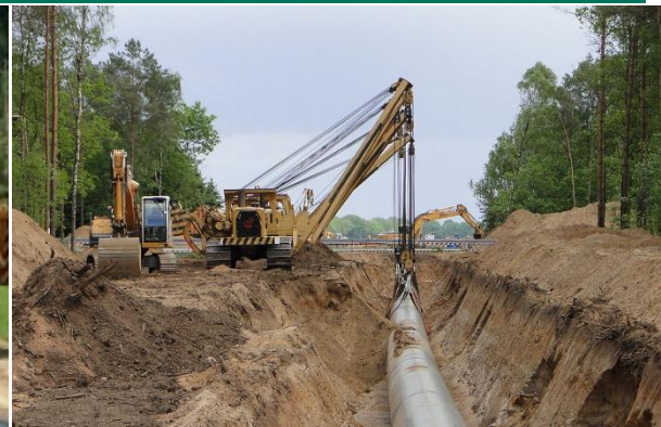
Final placement of a pipeline along a newly created corridor through a wooded area
