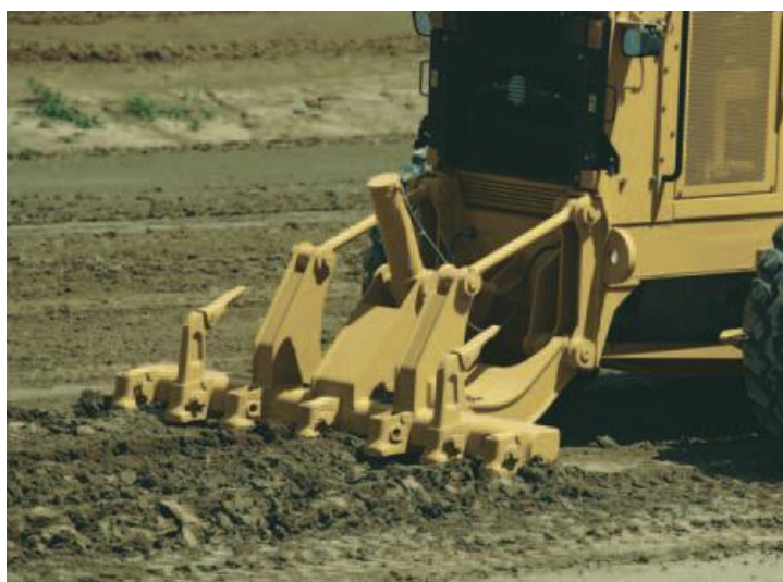
Figure 26: Grader ripping compacted soil.
