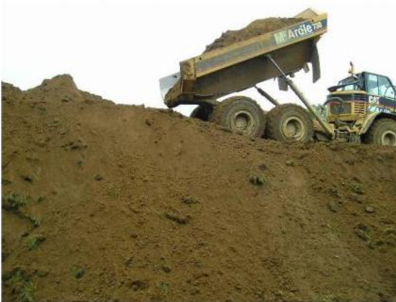
Figure 24: Stockpiling topsoil.
