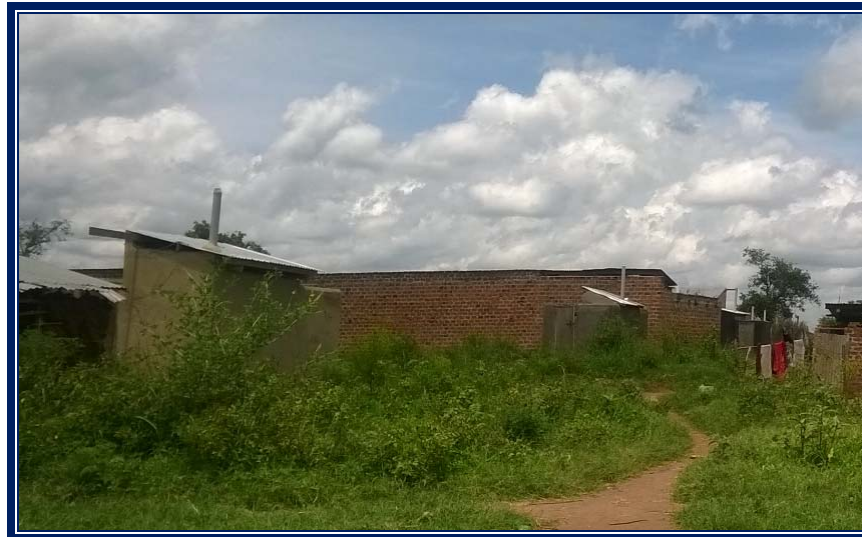
Figure 29: Vented improved pit latrines in Kyarushesha
