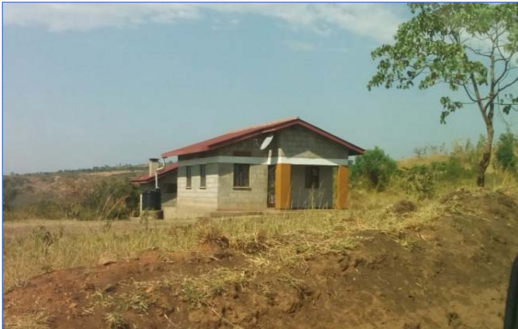
Photograph 16: Typical replacement house that will be built by CUL for resettled families on the Buhuka Flats
