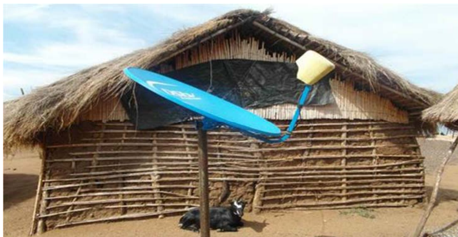
Photograph 2: A grass-thatched house in Busigi constructed with mud and wattle
