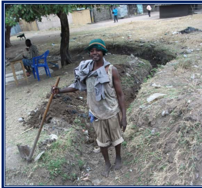
Figure 21: Clearing drainage ditches
