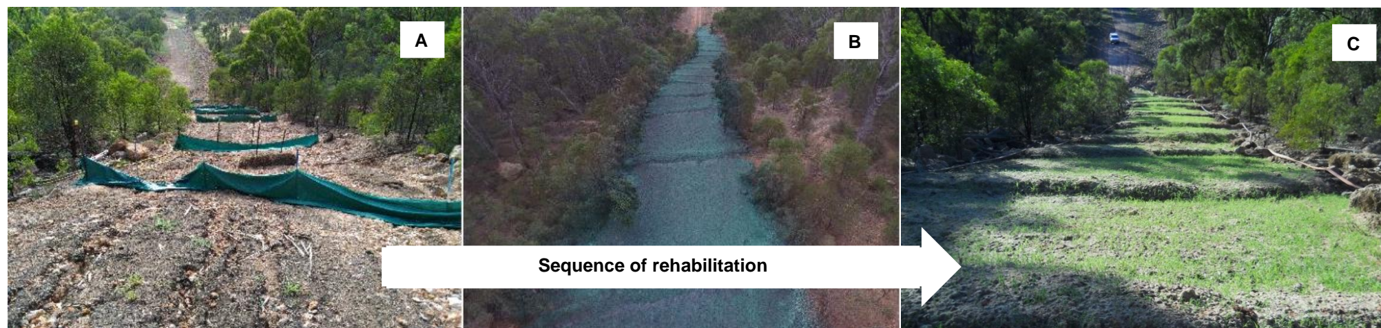
Figure 4: Rehabilitation of a backfilled pipeline corridor (Beneterra, 2017. [Online] Available: https://www.beneterra.com/beneterra-completes-difficult-pipeline-corridor-rehab/ ).
