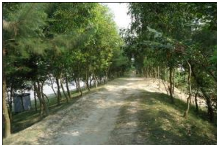
Typical road side plantation on embankment
