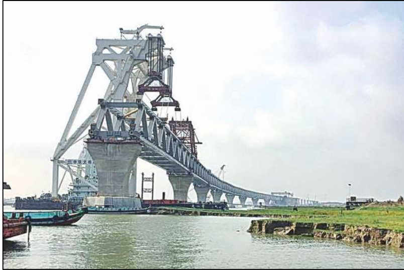
Padma bridge under construction
