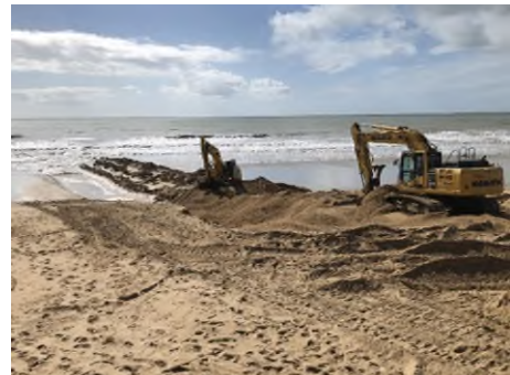
Photo : Fight against erosion for the landing of the DUNANT marine cable on the beach of Saint-Hilaire de Riez (France) source: https://merceron.com/
