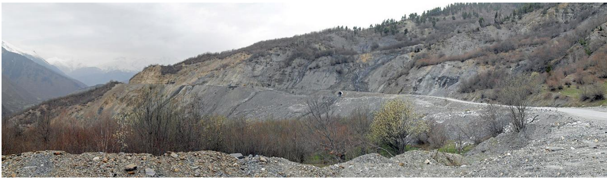
Photo 17. Instable mountain slopes above newly constructed road
