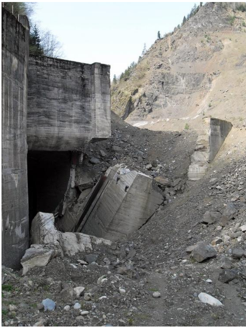
Photo 13. Collapsed inlet of river diversion tunnel
