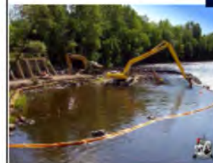
Application of silt screens in dredging operations
